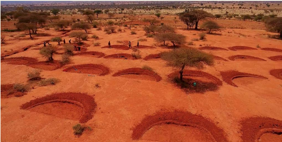
Figure 7: Semi-circular water bunds in Tanzania that capture runoff water and increase infiltration [image: Justdiggit]
